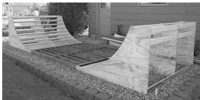
Frames put together before attaching the decking.
